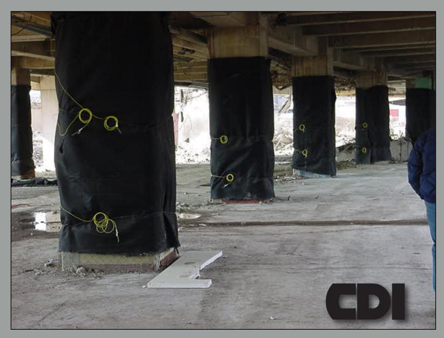
This is just one floor of a properly rigged building (by Controlled Demolition, Inc.) prior to demolition. A similar process would have been necessary to properly wire and demolish the Twin Towers. It's patently absurd to think that dozens of technicians, or more, were involved in any normal demolition process. The Twin Towers were not destroyed by standard demolition practices. This was a nuclear event and the dust and elements within the dust prove this beyond any doubt.
